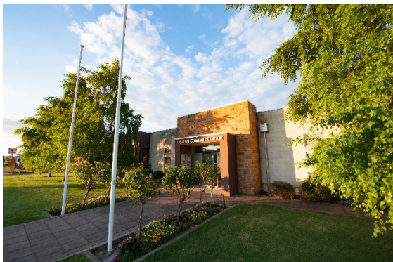
District Council of Grant Principal Office
